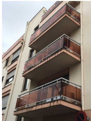
PMMA from deconstruction
